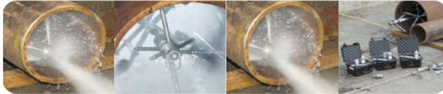
RETRO JETTING DEBRIS PIPE CLEANING PROCESS
