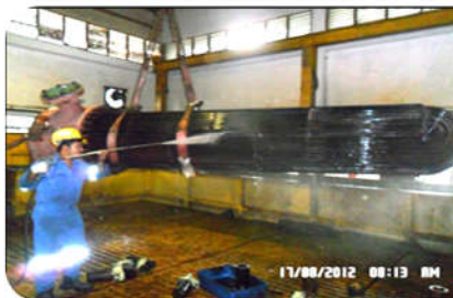
HEAT EXCHANGER HIGH PRESSURE WASH
