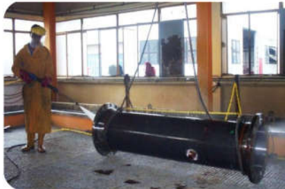
HIGH PRESSURE WASH
