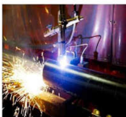
PIPE MACHINE WELDING
