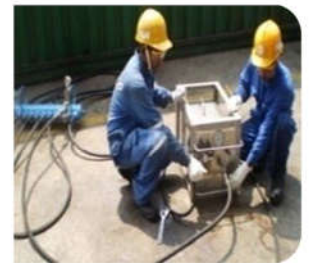
PRESSURE TESTING PROCESS
