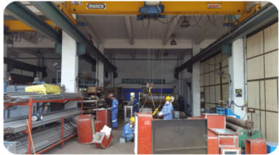
HVAC FABRICATION WORKSHOP
