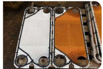
HEAT EXCHANGER PLATE BEFORE & AFTER CHEMICAL CLEANING
