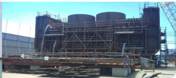
HANDLING NEW FPSO MODULES & SUPPLY VESSEL
