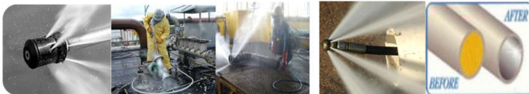
WATER JETTING PROCESS AND PIPELINE JETTING PROCESS
